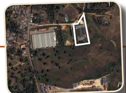
▲ Aerial photograph with plot layout and positioning.
